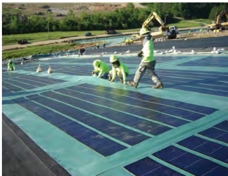
Landfill Capped with Solar Panels to produce energy on 'wasted' land.
